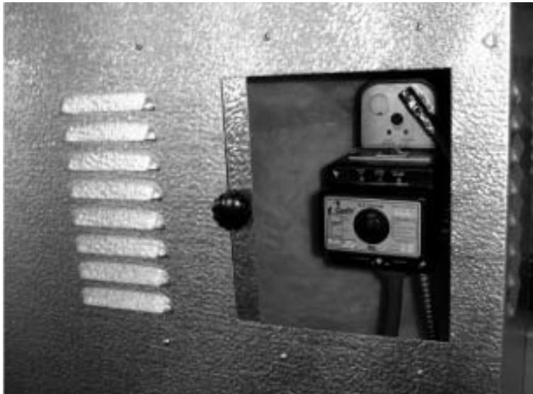
Slide panel allows for easy access to the boiler control. Pool temperature is set using a dial located at the bottom of the control on the outside of the box.
